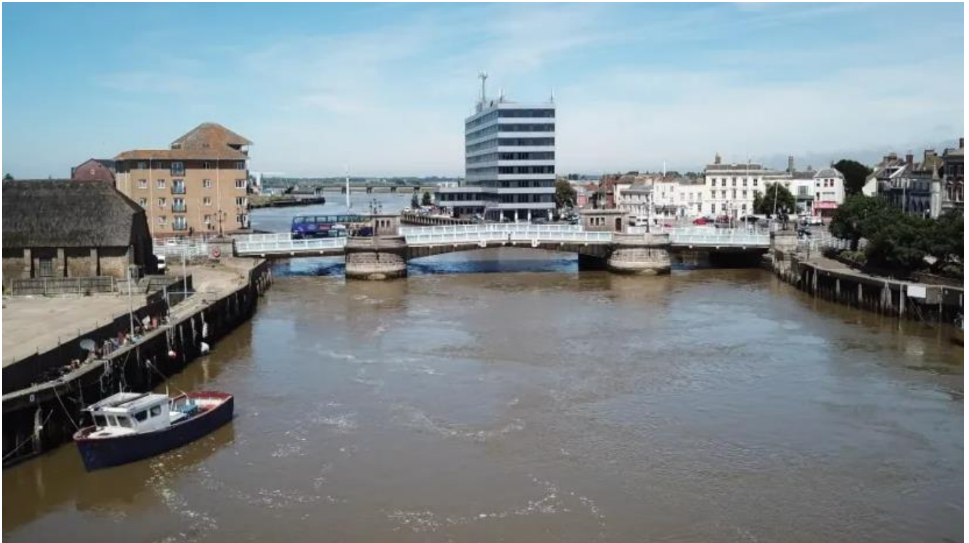
Haven Bridge viewed from SE (seaward)
