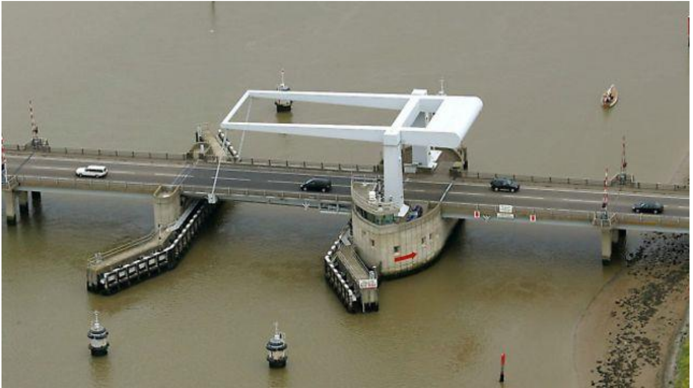
Breydon Bridge viewed from W (note side-spans on either side of lifting span)
