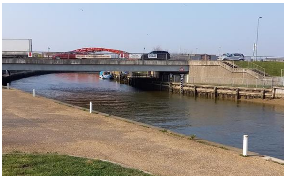
Acle Road Bridge viewed from N (upstream)
